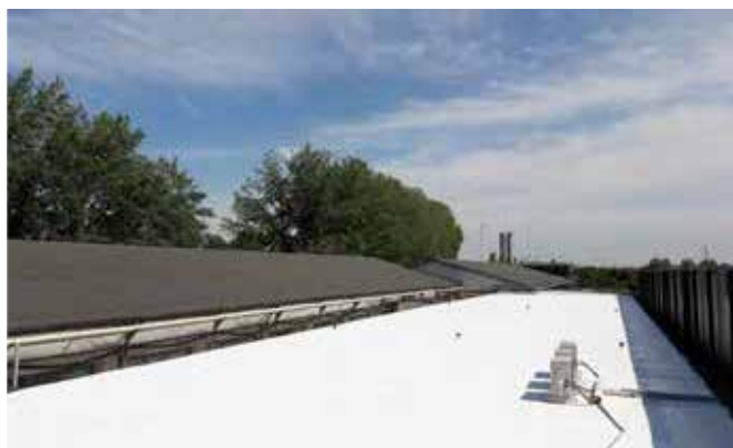
Fig. 2. The view of reflective waterproofing roof coating COOL-R produced by Libra Sp. z o.o
