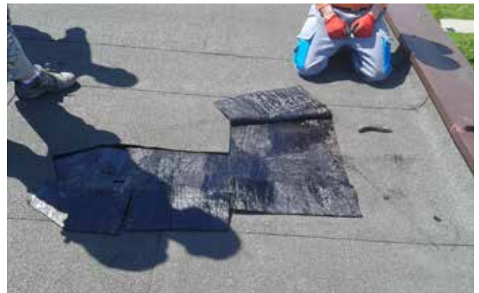
The substrate inspection. Air blisters removal
