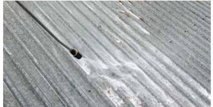
Roof washing - active foam
