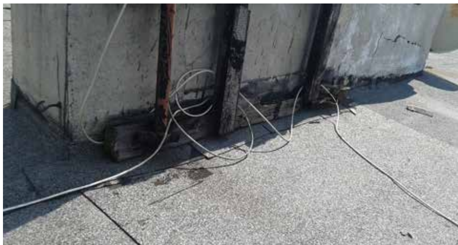
Elements to be removed before the application of COOL-R
