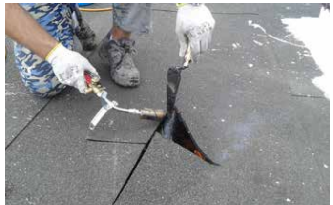
Substrate repair
