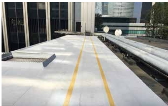
Example maintenance path
