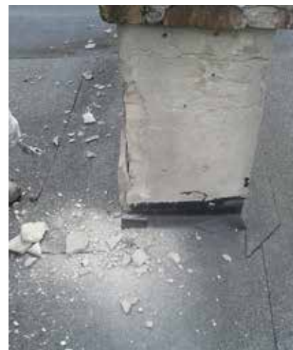
Blistered pattern on a chimney
