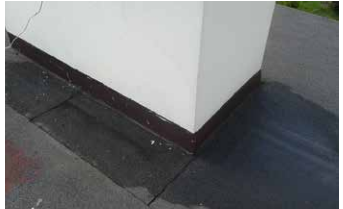
Moisture on the substrate after washing
