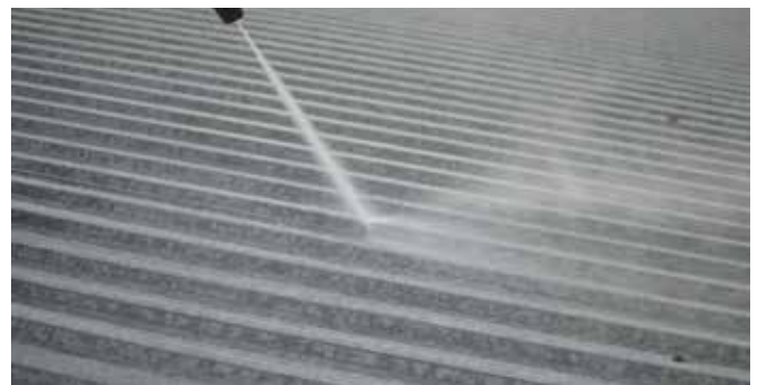
Roof washing - rinse the active foam with clean water
